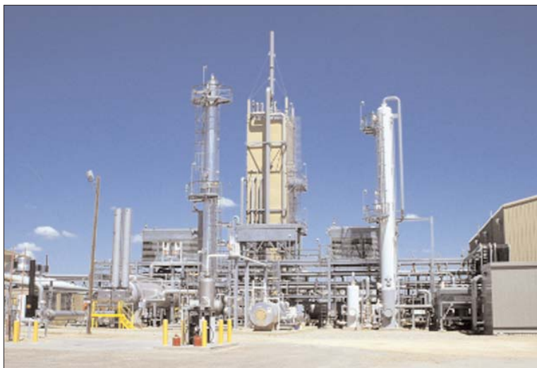
The Crude Helium Enrichment Unit (CHEU), which separates the natural gas, helium, and other byproducts out, came online in 2003 and is operated by BLM in partnership with the CRLP. Photo courtesy of BLM.
